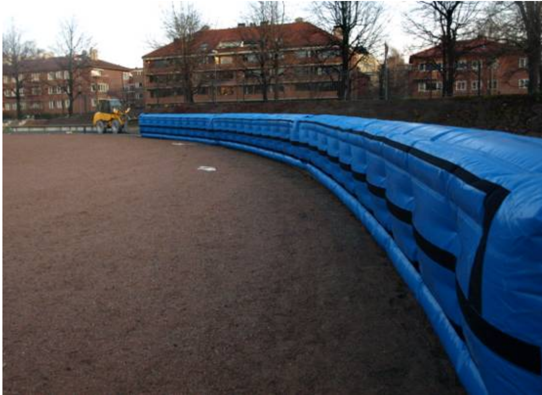
Second reference in progress, Frogner Stadion, Oslo
